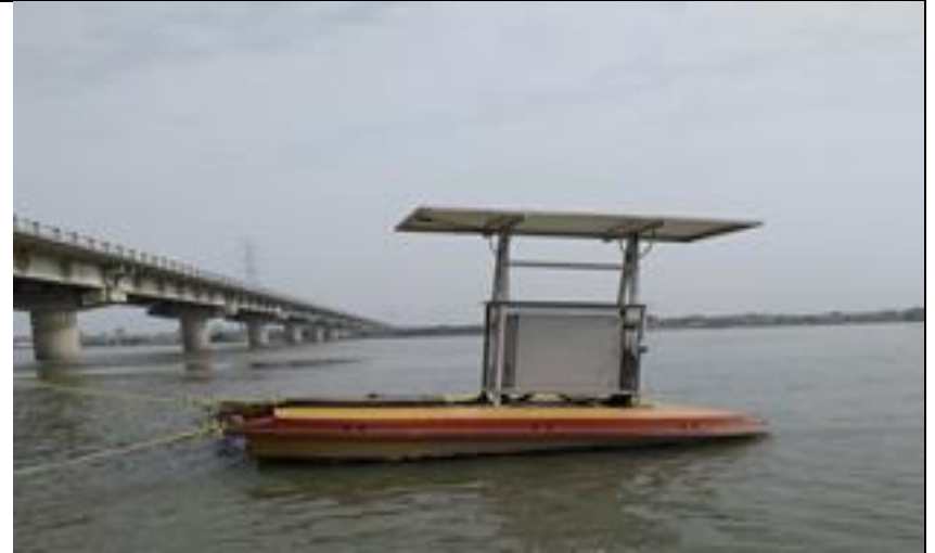
Bithoor Bridge, Kanpur (UP-18)
