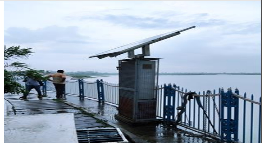
Barrage at Kanpur (UP19)
